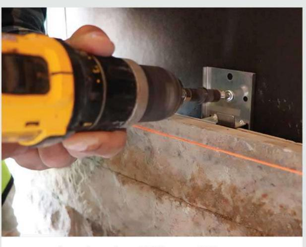
A galvanized Clip and Screw mechanically fastens the product to the wall, eliminating the necessity of a traditional mortar and wire lath installation.
