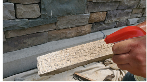
NO EXISTING SCRATCH COAT ON STONE
