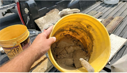
POLYMER MODIFIED MORTAR
