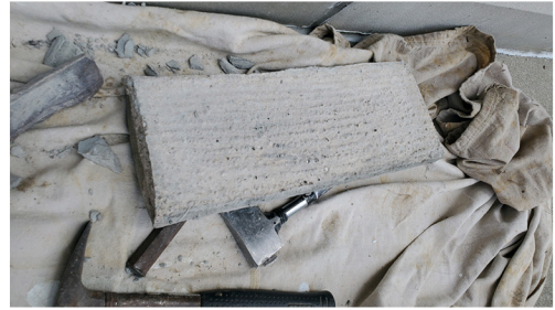
NO EXISTING SCRATCH COAT ON STONE
