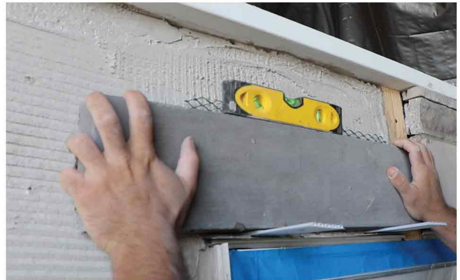
Attaching the Lintel
