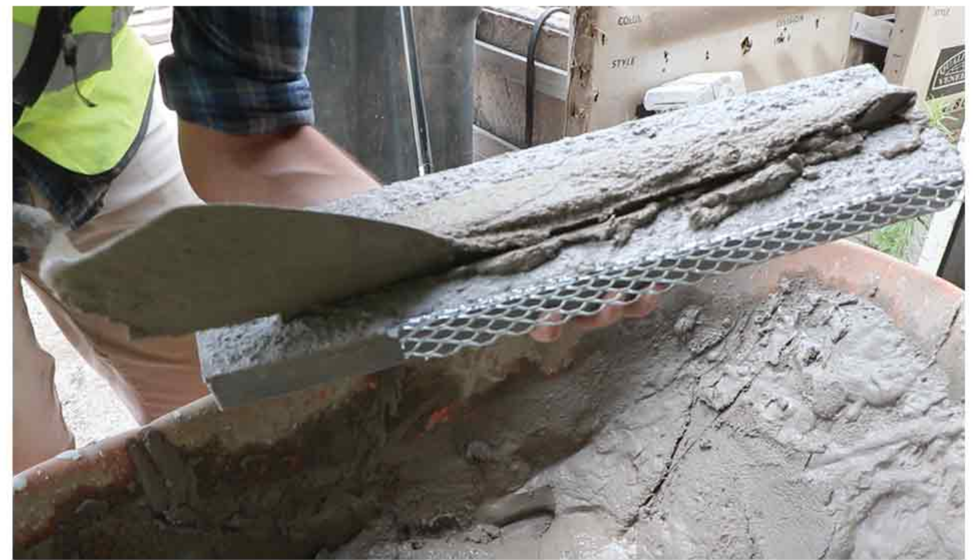
Leveling the Lintel
