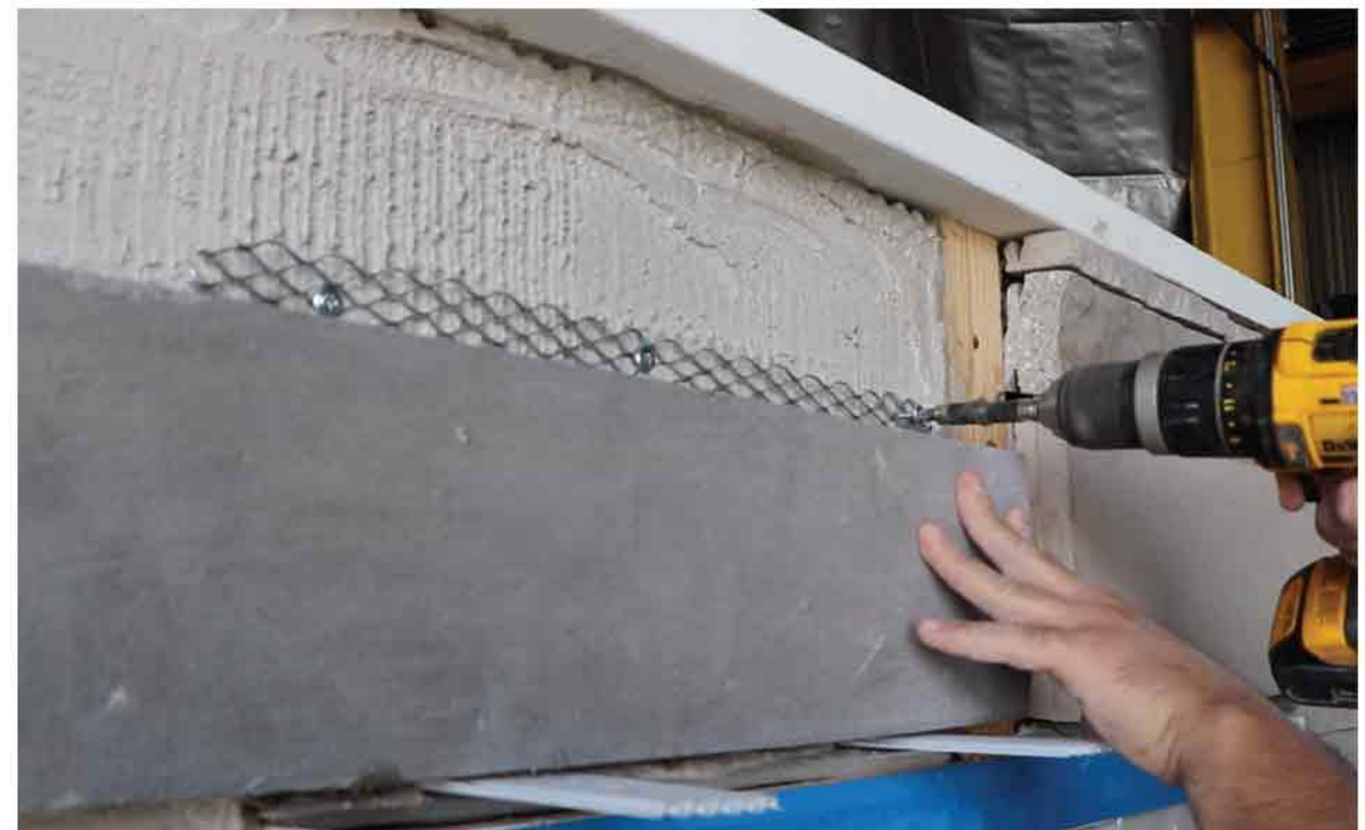
Attaching the Lintel
