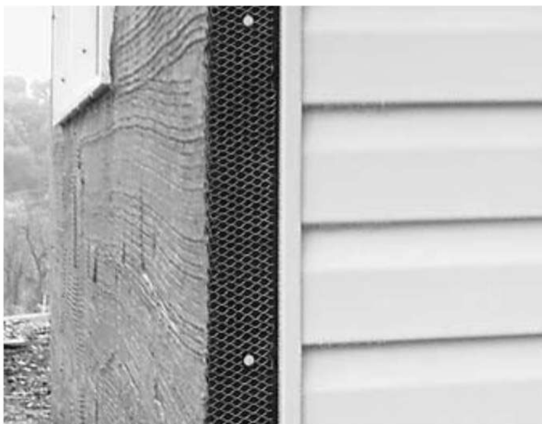
Fig. 3 Wrap the lath around corners.
