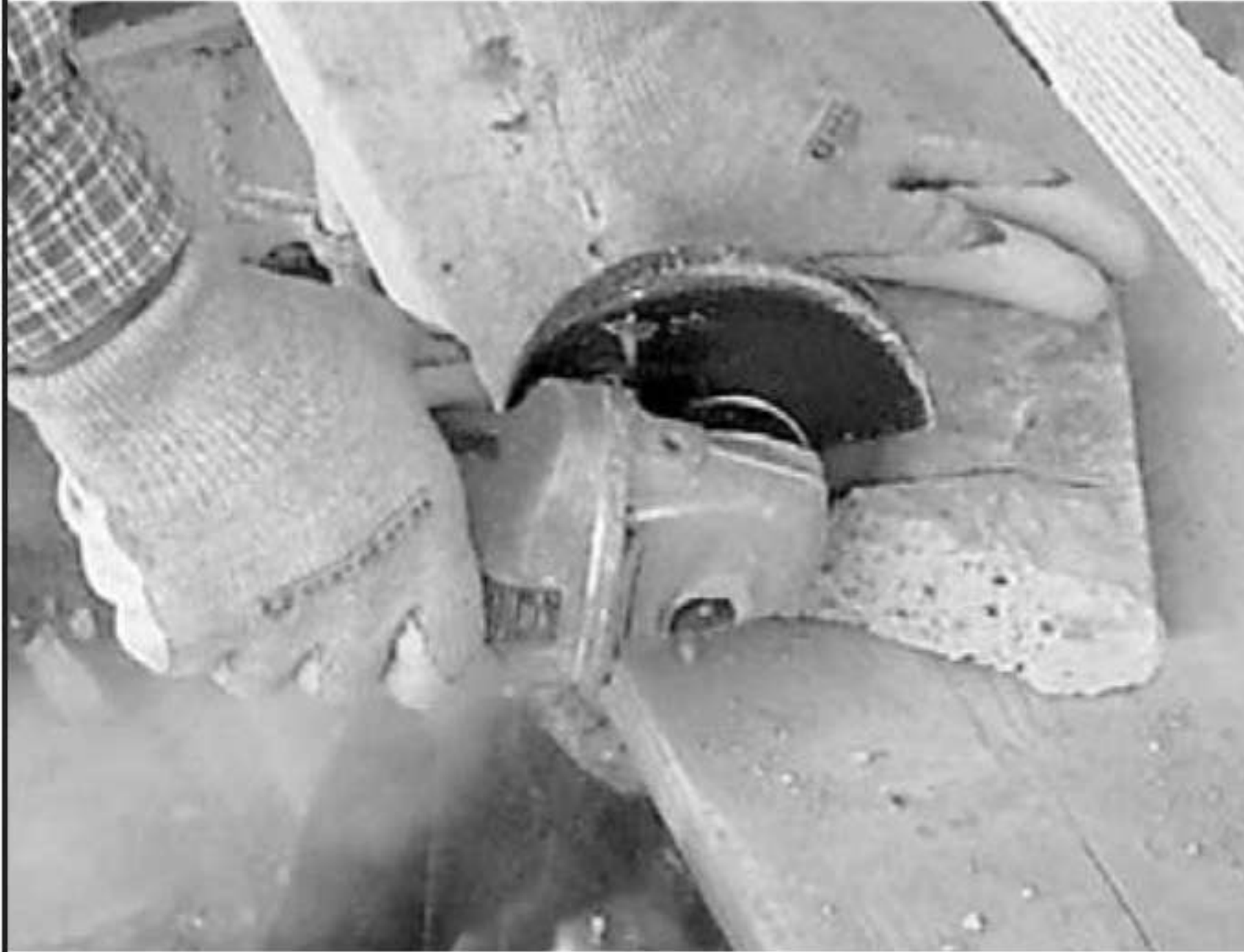
Fig. 7 Trimming the stone.
