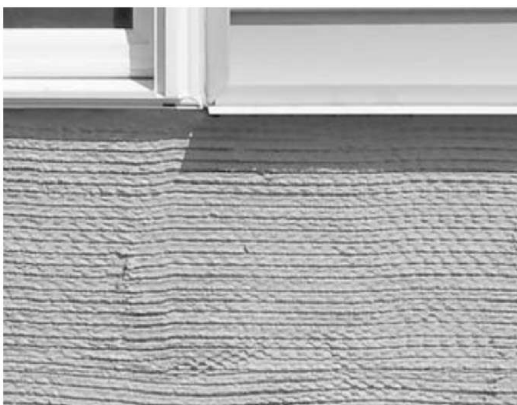
Fig. 4 Apply the scratch coat over the lath.
