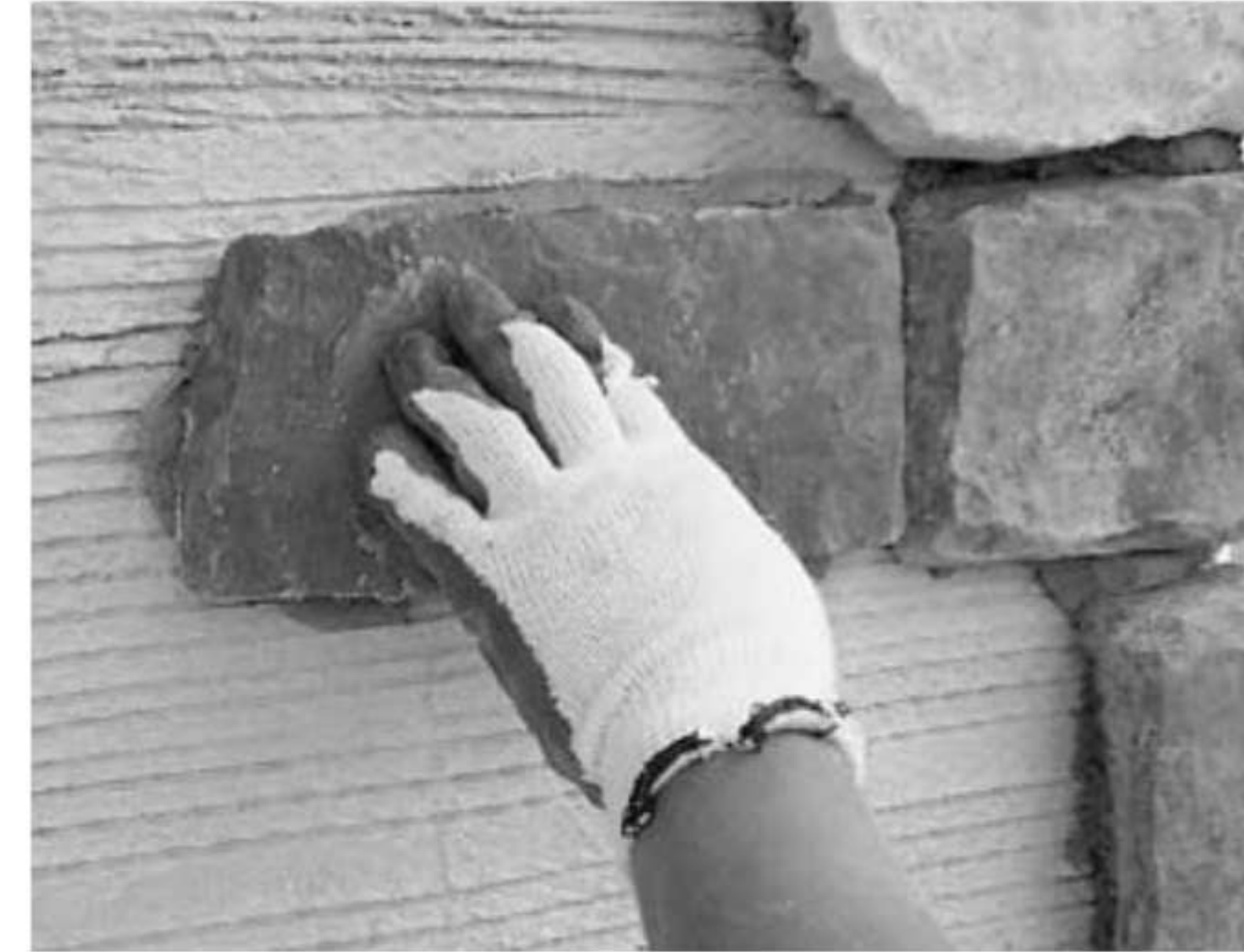
Fig. 9 Setting the stones.
