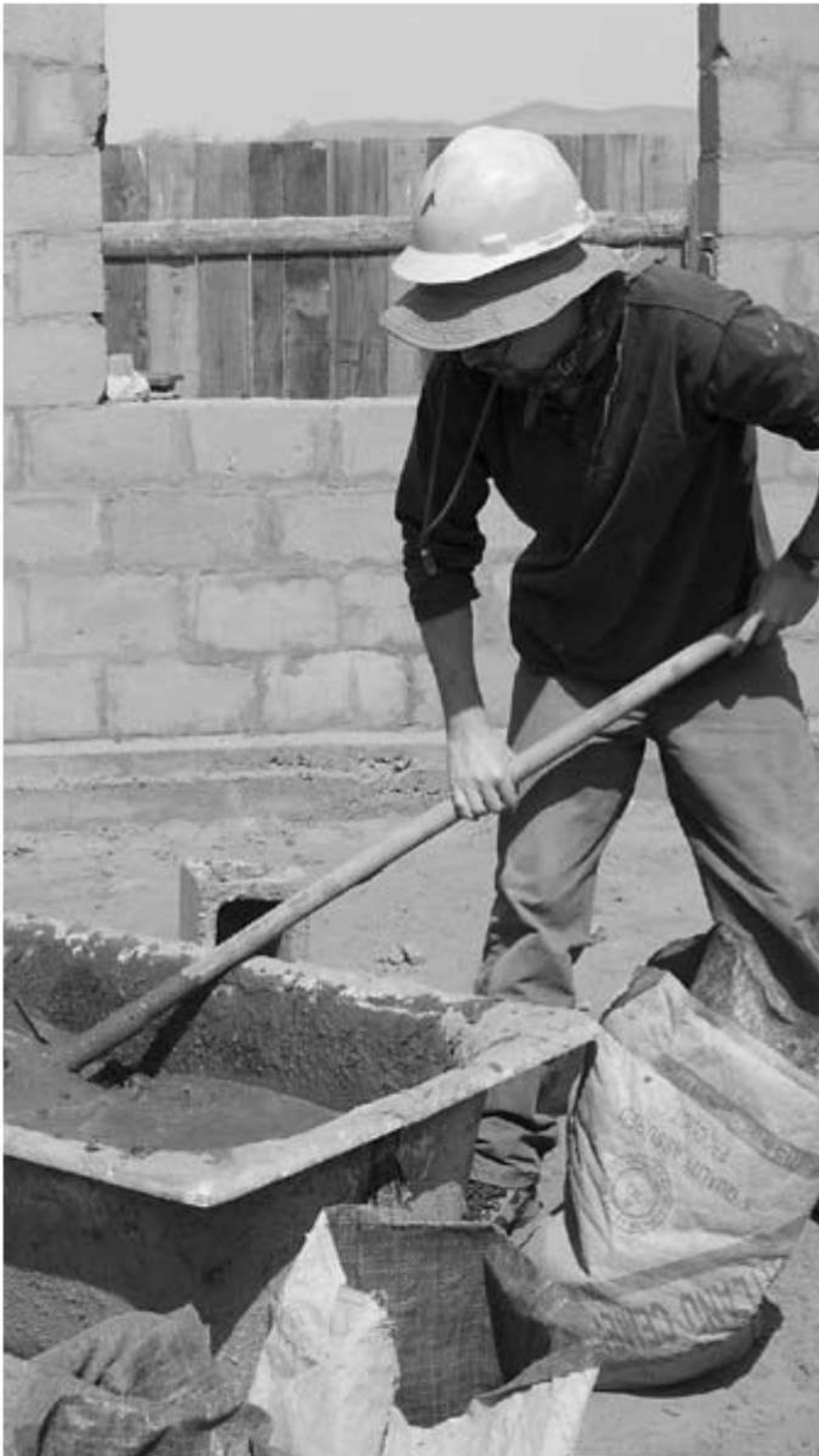
Fig. 6 Mixing the mortar.
