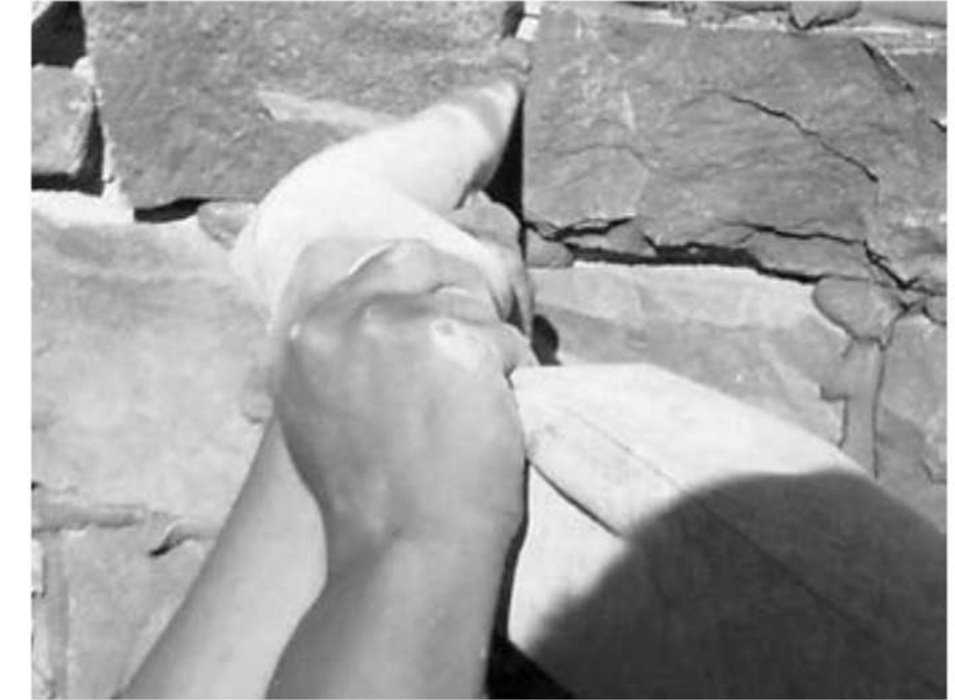
Fig. 10 Grouting the stones.
