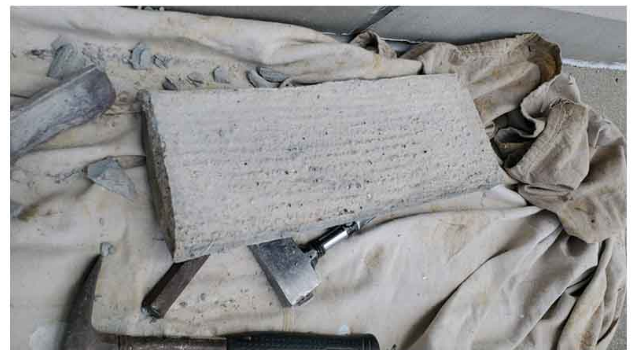
REMOVE ANY EXISTING MORTAR FROM STONE
