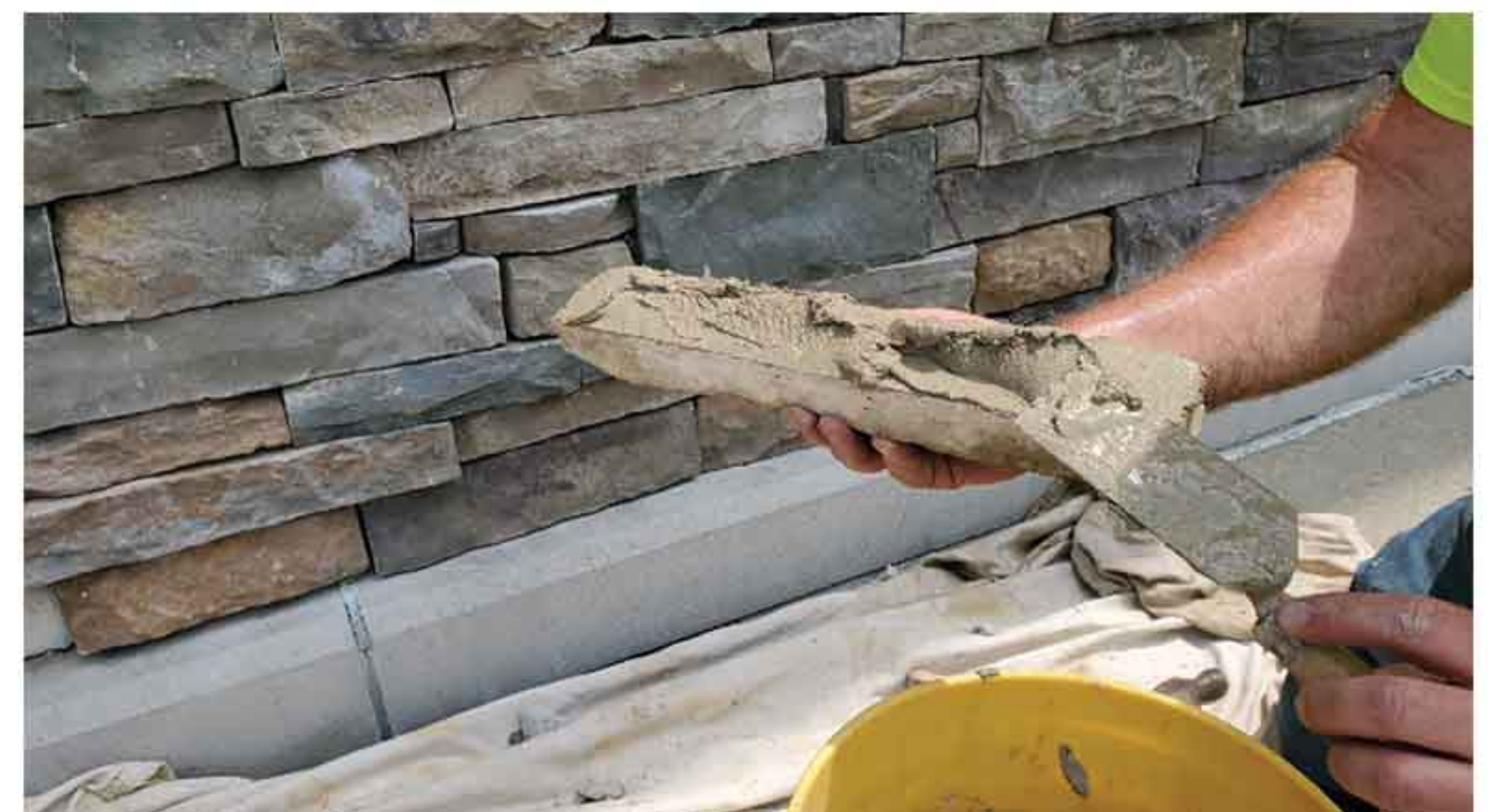
FULL MORTAR COVERAGE ON BACK OF STONE
