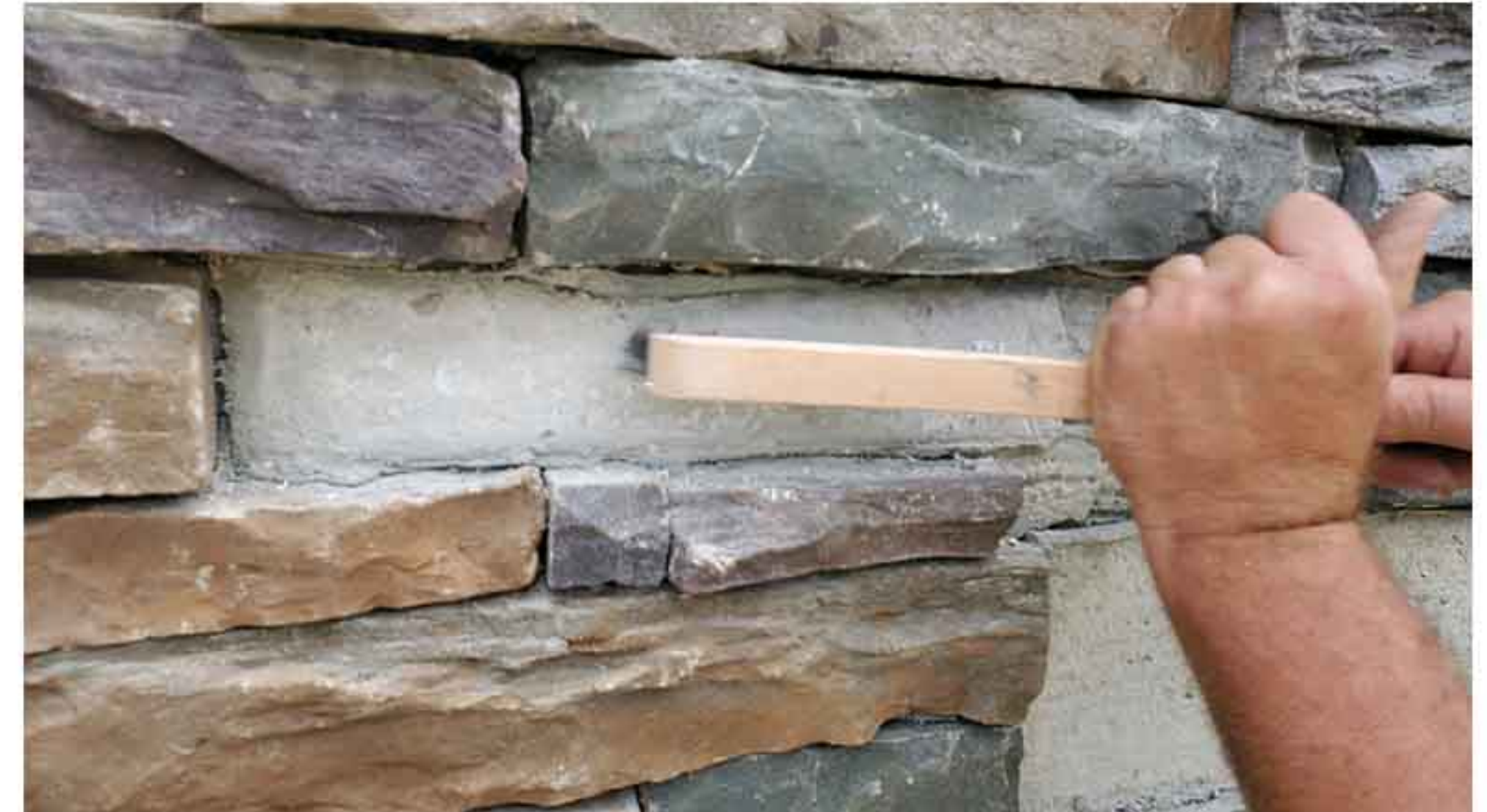
WIRE BRUSH CLEANING TO SCRATCH COAT
