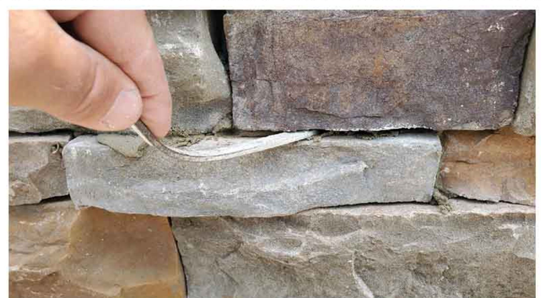
REMOVE EXCESS MORTAR
